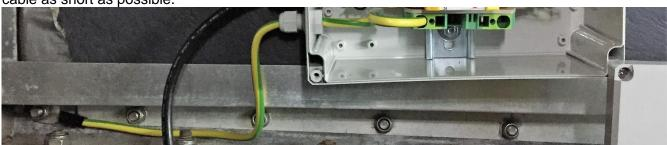
3. Cut the WSS sensor cable and strip off about 5 cm. Fold the screen backwards leave approximately 2 cm of screen and cut the access screen. Insert the cable end into the earthing spring. If necessary secure the cable in the spring with zip ties.
