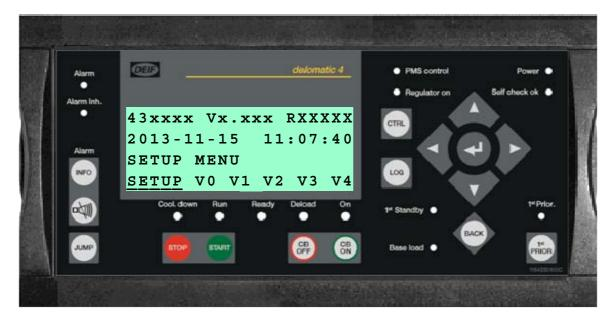
The window above shows the project number, software version and release in the first line, the date and clock in the second and the text SETUP MENU in the third line. In line four, it is possible to select the SETUP menu or V0-V4:
